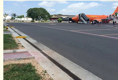
ACO Airport drainage systems https://www.aco.co.za/products/airport-drainage-systems
